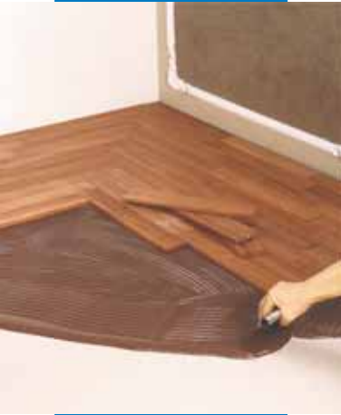
Applying the adhesive with a notched trowel for wood
