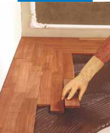
Installing a 14 mm Teak plank
