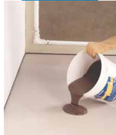
Pouring the adhesive onto the screed
