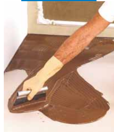
Applying the adhesive
